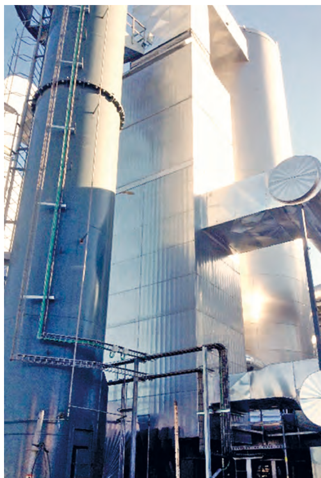
Bottom · Preheater gas recirculation outlet of the boiler Source: E&M Combustión
